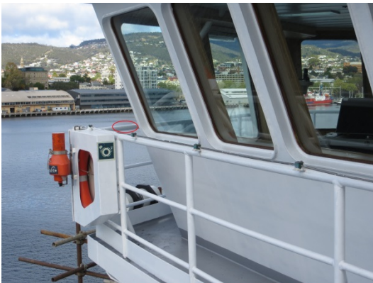
Figure 2: KT15 radiometer (top left), U-shaped attachment for attaching to railing (top right) and approximate proposed location for KT15 installation on RV Investigator marked with red ellipse (bottom).
