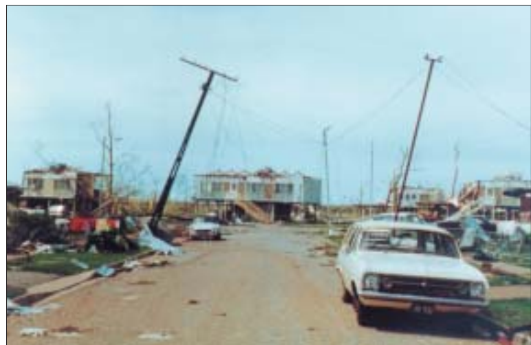
Damage caused by tropical Cyclone Tracy in Darwin – December 1974. Image courtesy of the Bureau of Meteorology
