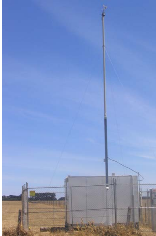
Figure 2. Atmospheric monitoring module and tower.
